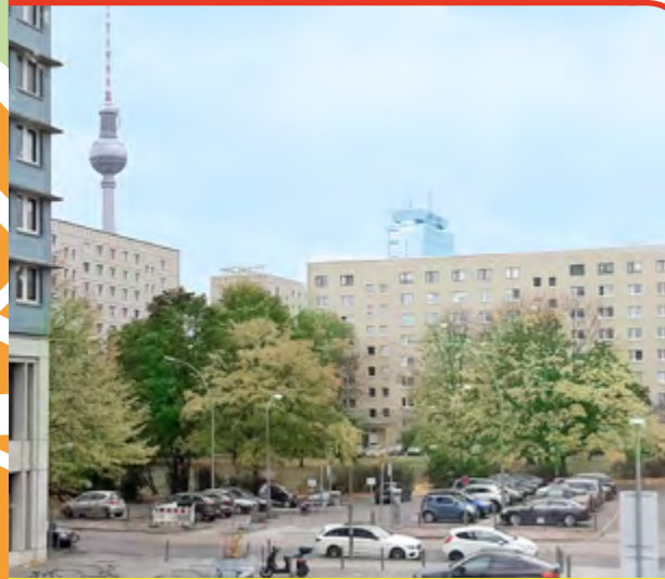
Building Site Berolinastraße
